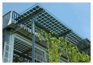
Figure 9 Integrated PV in shading structure
